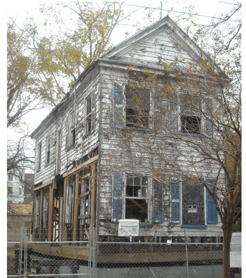
83 Nassau Street under construction
