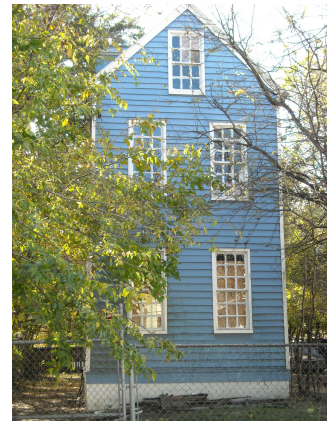
89 Nassau Street property to be renovated into 4 studio apartments.
