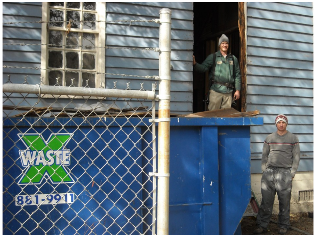
Palmetto Craftsmen Construction workers beginning renovations on the 89 Nassau Street property.
