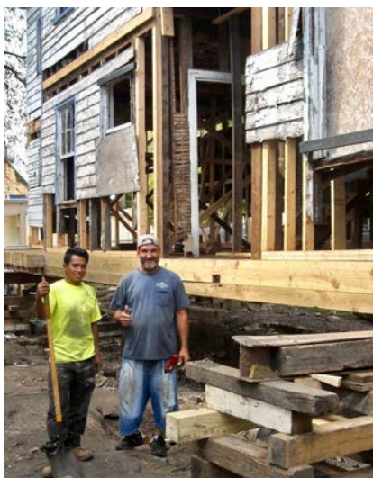
83 Nassau Street house being lifted above floodplain.
