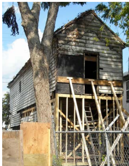
Stabilization work being completed on 83 Nassau Street.
